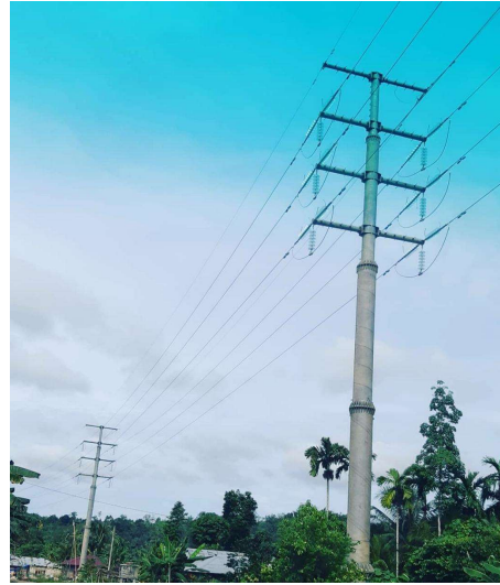
Gambar 2.9 Steel Pole
